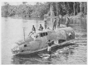
**5** Floating on a raft of logs, forward part of fuselage begins trip to shipping port; souvenir hunters sometimes strip valuable data from crashed Jap planes which are needed so American pilots can get information on firepower, flight characteristics
